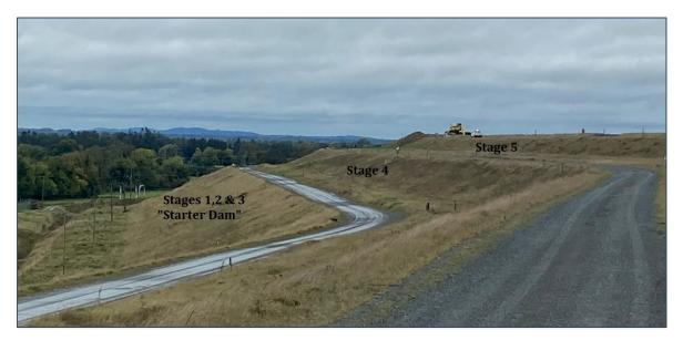
Plate 13.1: Existing embankments side profile (provided by the client)
